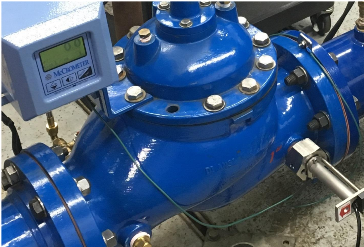
Figure 26: Converter & probe with ground wiring
